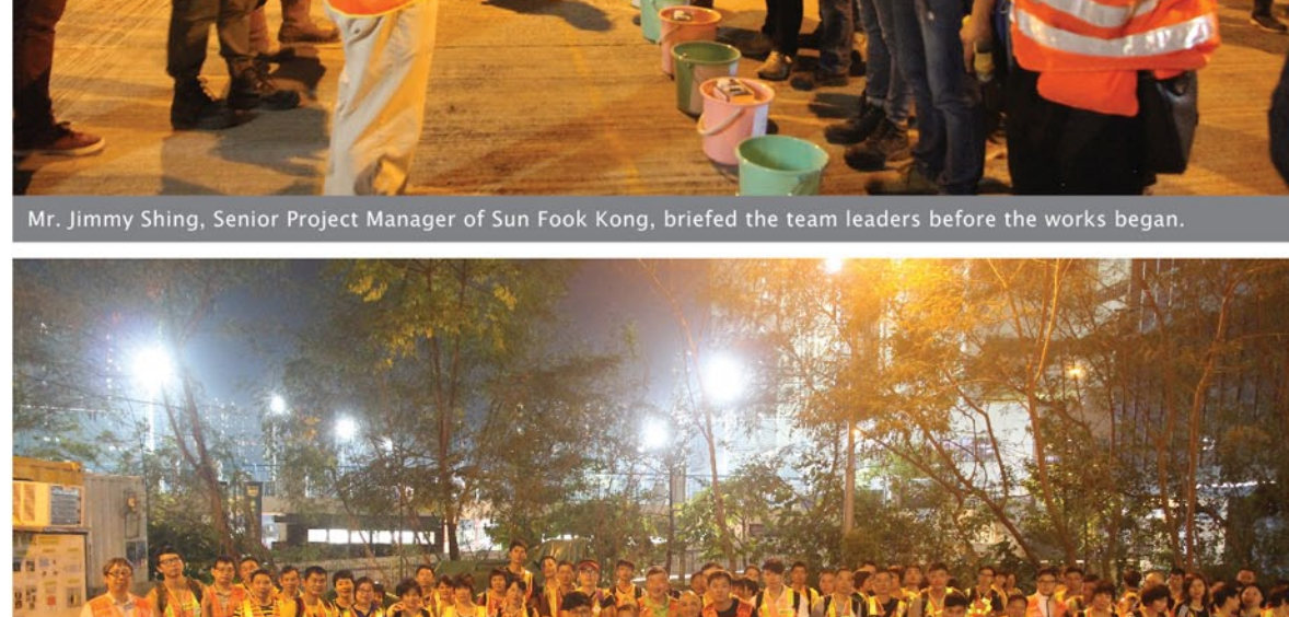
Mr. Jimmy Shing, Senior Project Manager of Sun Fook Kong, briefed the team leaders before the works began.
